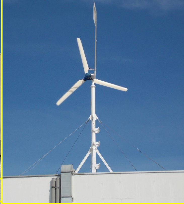
1,4 kW wind turbine on the roof
