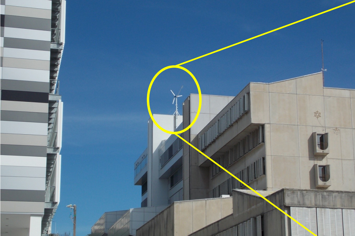
1,4 kW wind turbine on the roof
